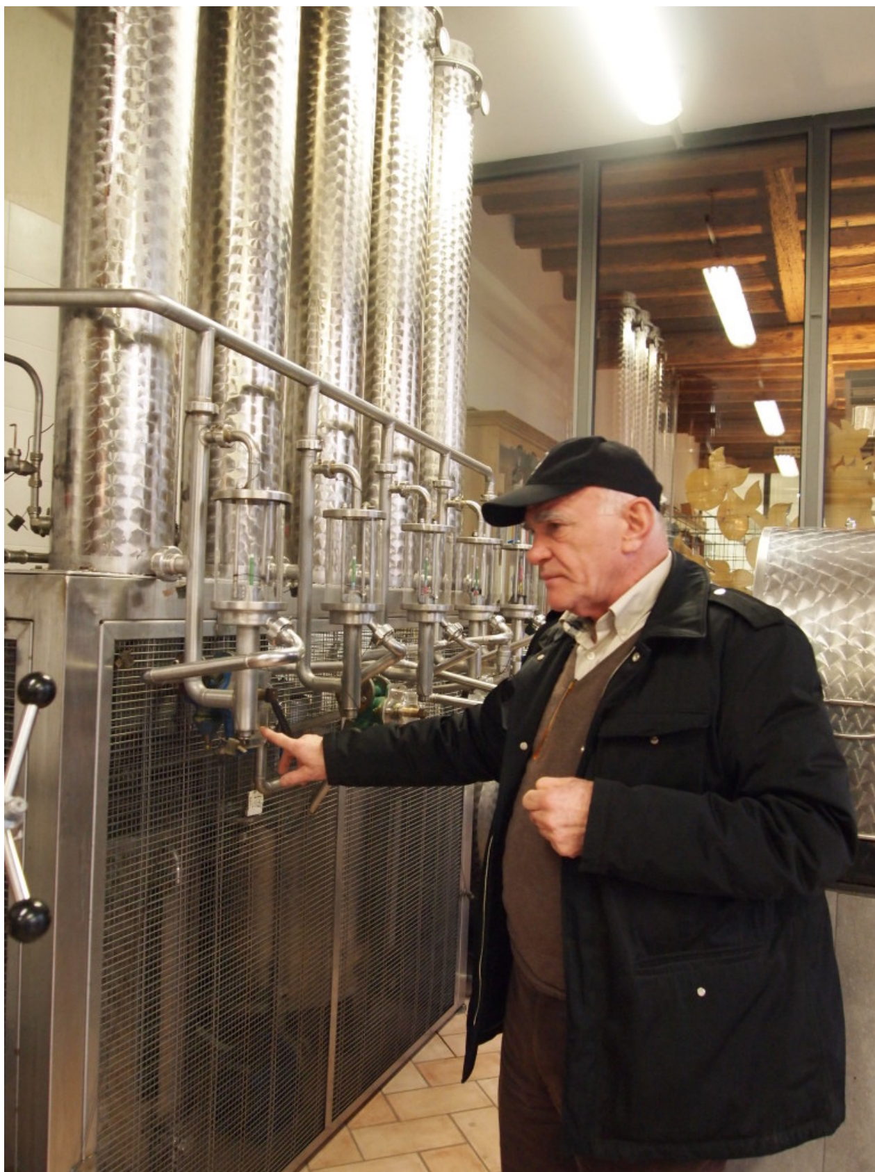
Distilleria Capovilla – Interni
